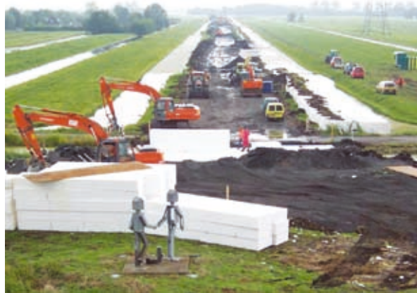
Figure 39: Building a road on EPS (polystyrene)
